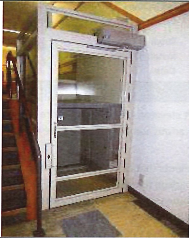
Main Hall Entrance
